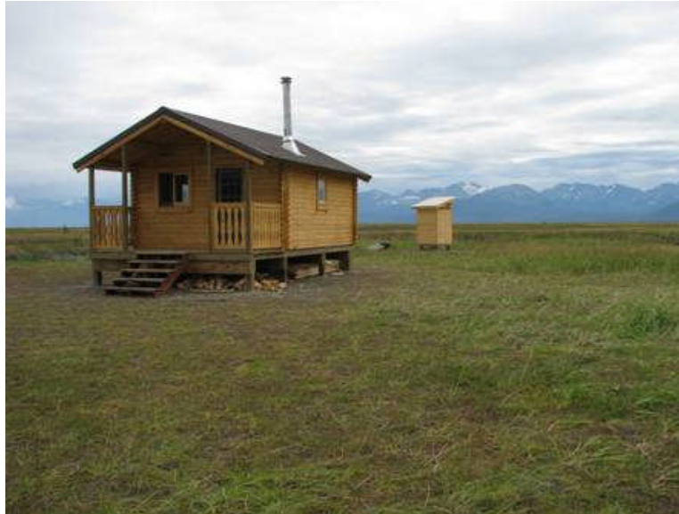
Figure 7. Pincher Creek cabin.
