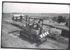
BULLDOZER OPERATING IN L 1 -5,-6,-7,8 DURING JUNE.
