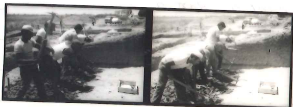
WORK IN PROGRESS, PROCEEDING NORTHWARD
