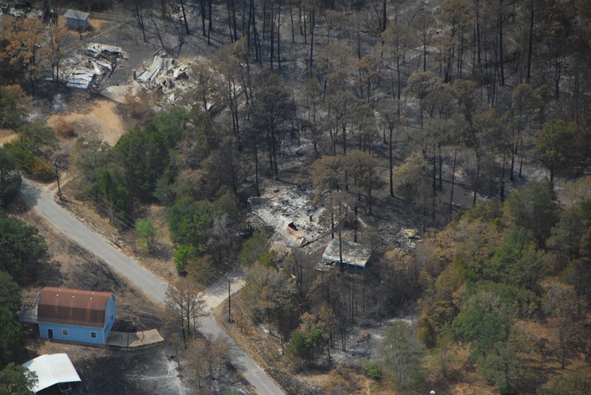
Another well-composed view of intact and destroyed homes near the fire perimeter.
