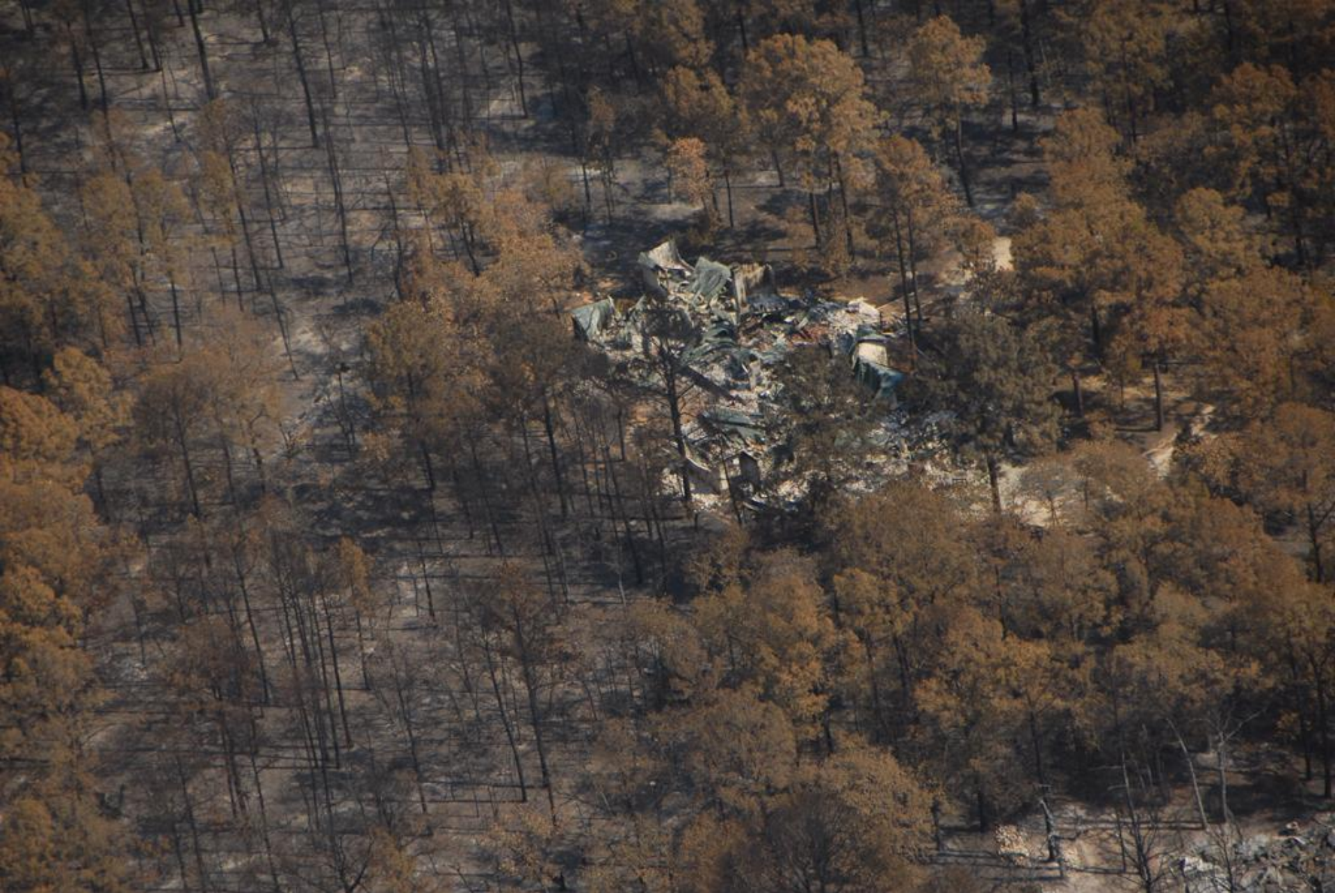
An exceptionally detailed view of damage to an individual residence.
