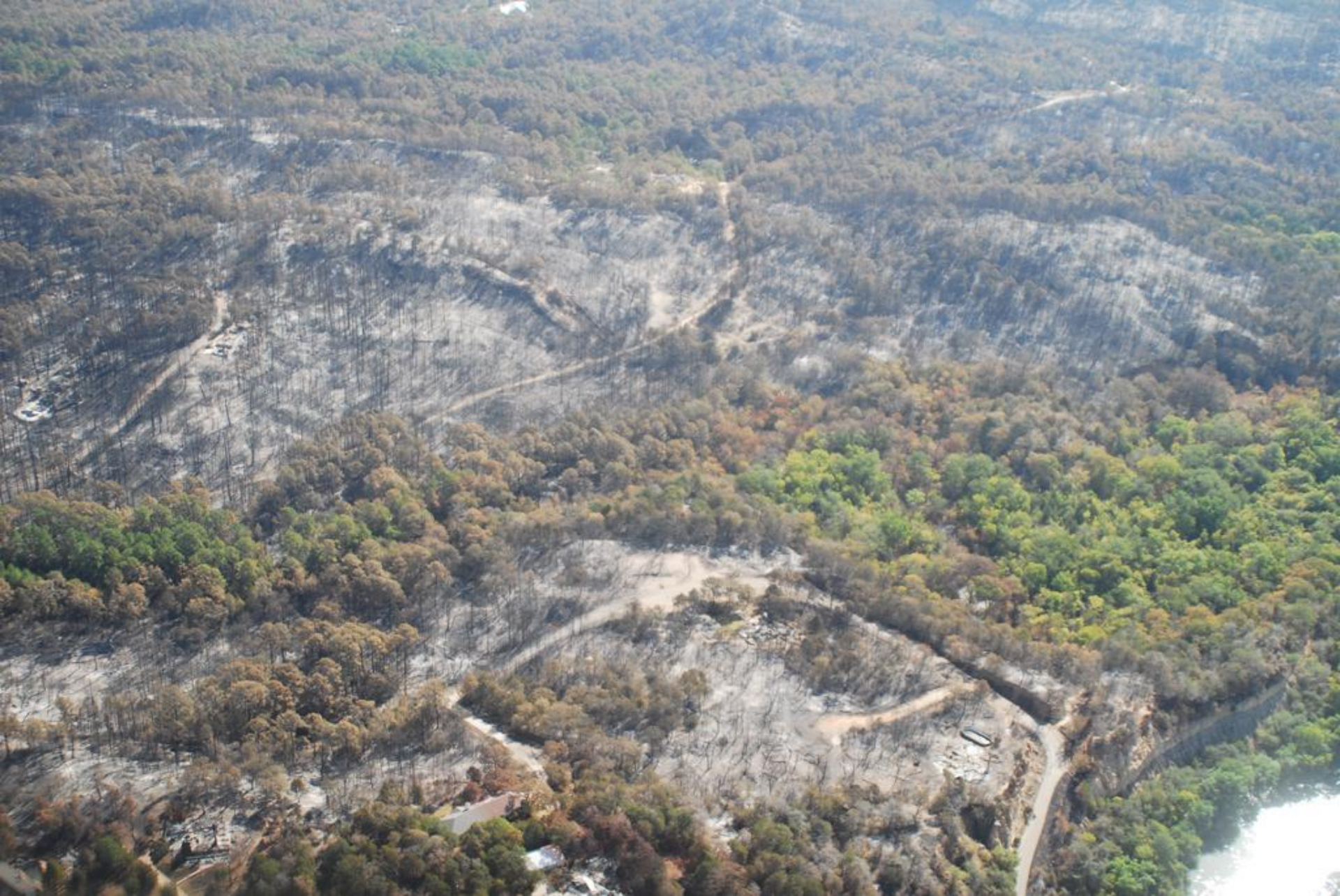
Very good low oblique view of damaged structures under excellent illumination conditions.
